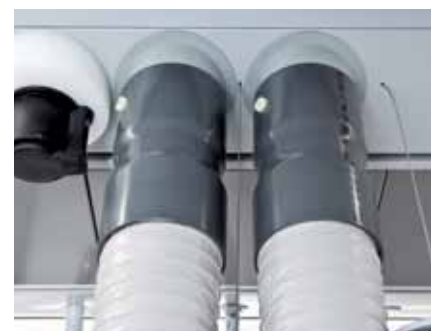
Exhaust air connection of the AeroEm to the Service Wing.
