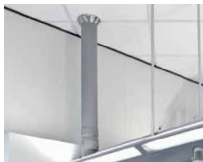
Exhaust air connection of the Service Wing.
