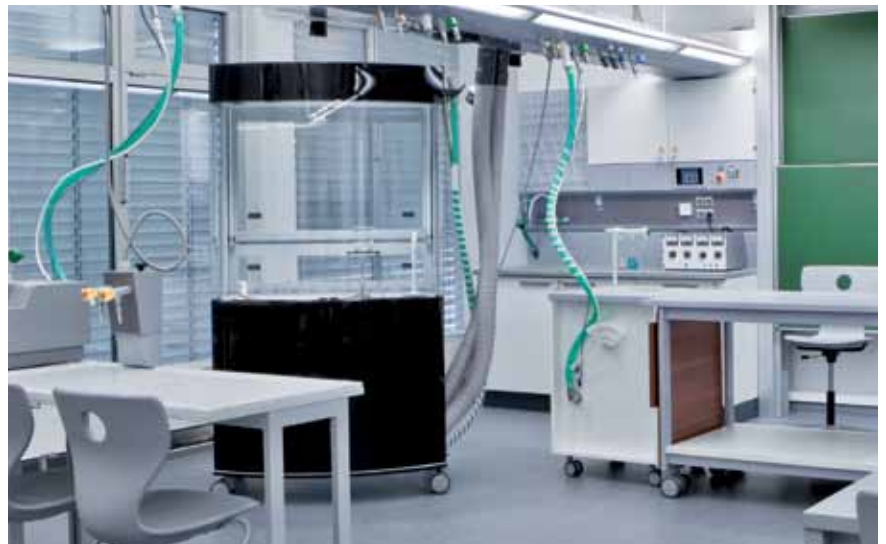
Exhaust air connection of the Service Wing.
